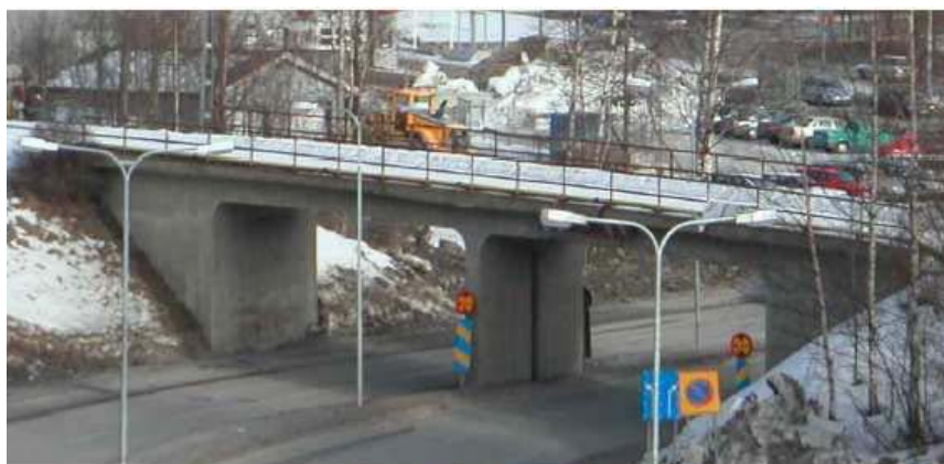
Fig. 1: Örnköldsvik Bridge (Elfgren et. al., 2007)
