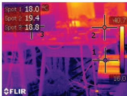
Fig. 2: Images taken by FLIR infrared camera
