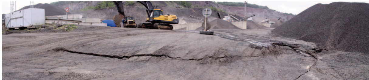
Fig. 3: Open cracks at the offices of the quarry Dobkovičky on the day before landslide
