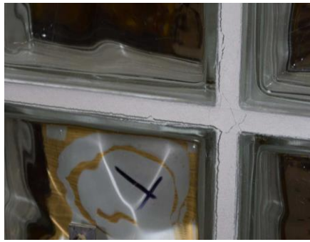
Fig. 7: Cracks in the joint.
