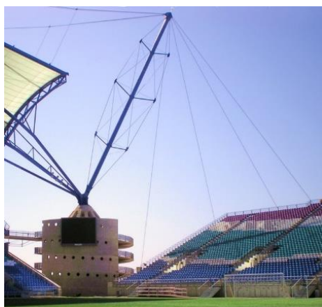
Fig. 1: Stayed column with 3 spaced crossarms (with 3 stays) supporting roof of Estádio Algarve Faro (left), planar stayed column (with 2 stays) supporting facade of a building in London (right).
