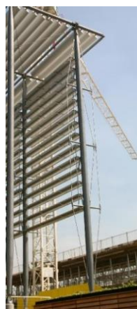
Fig. 1: Stayed column with 3 spaced crossarms (with 3 stays) supporting roof of Estádio Algarve Faro (left), planar stayed column (with 2 stays) supporting facade of a building in London (right).
