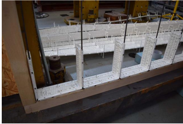
Fig. 2: The Vitralock system during the wall assembly.
