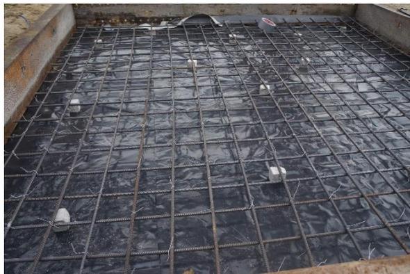
Fig. 5: Reinforcement – steel mesh.
