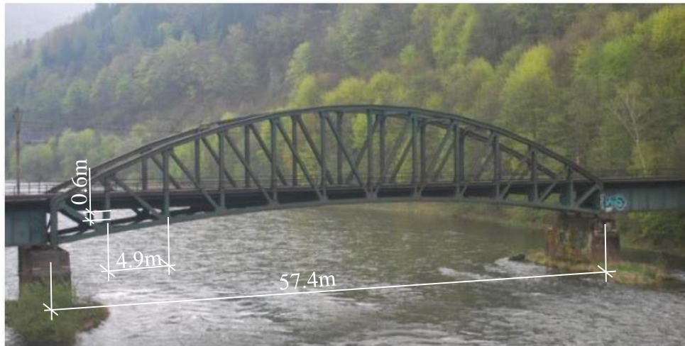
Fig. 2: Arch bridge over river Váh near Strečno.
