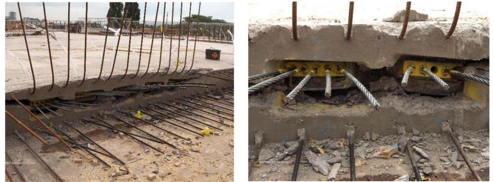
Fig. 2: Tendon failure at the end of the slab
