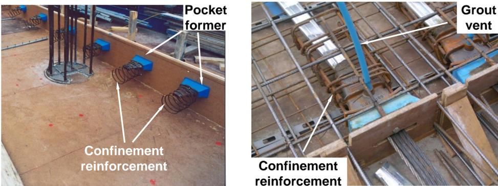
Fig. 1: Live-end anchorage with confining steel
