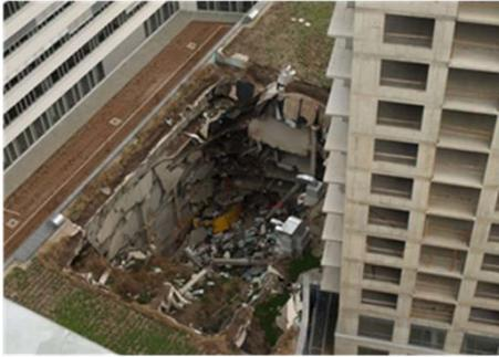
Fig. 1: Progressive collapse of a parking garage, Bratislava (2012).
