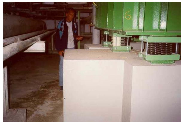
Fig. 2: Steel frame supported by spring units
