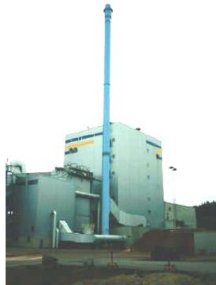
Figure 1 VEAB steel chimney
