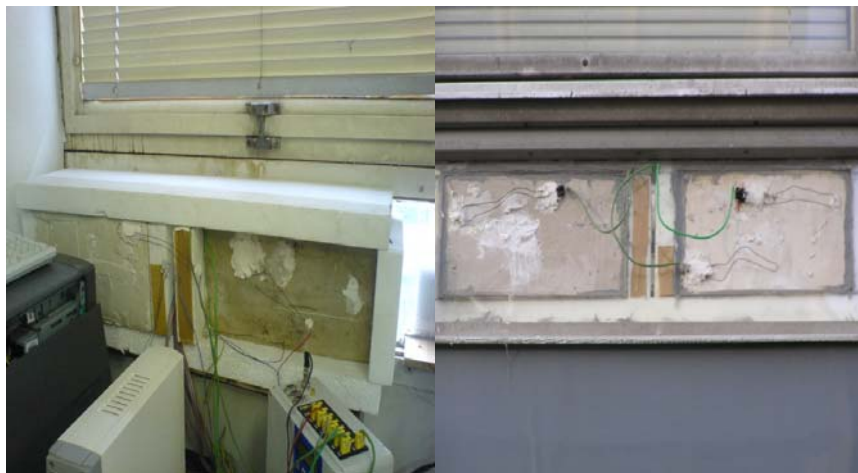
Fig. 1: The gypsum blocks (left – the interior side, right – the exterior side).
