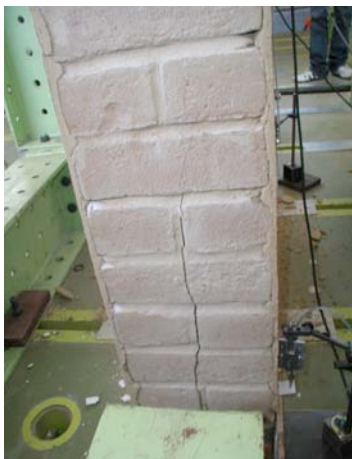
Fig. 13: Vertical crack in the wall thickness
