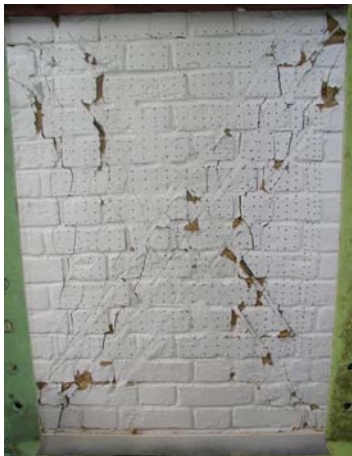
Fig. 9: Crack pattern at failure of the plain masonry control wall under a combination of vertical compression and cyclic shear.
