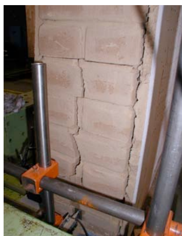
Fig. 11 - Evidence of the detachment of the plaster from the wall surface.
