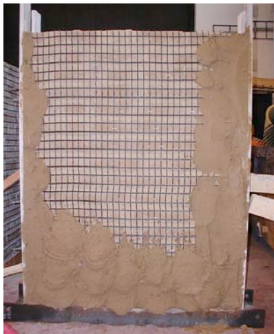
Fig. 2: Adobe brick wall with geo-nets (ABW_3)
