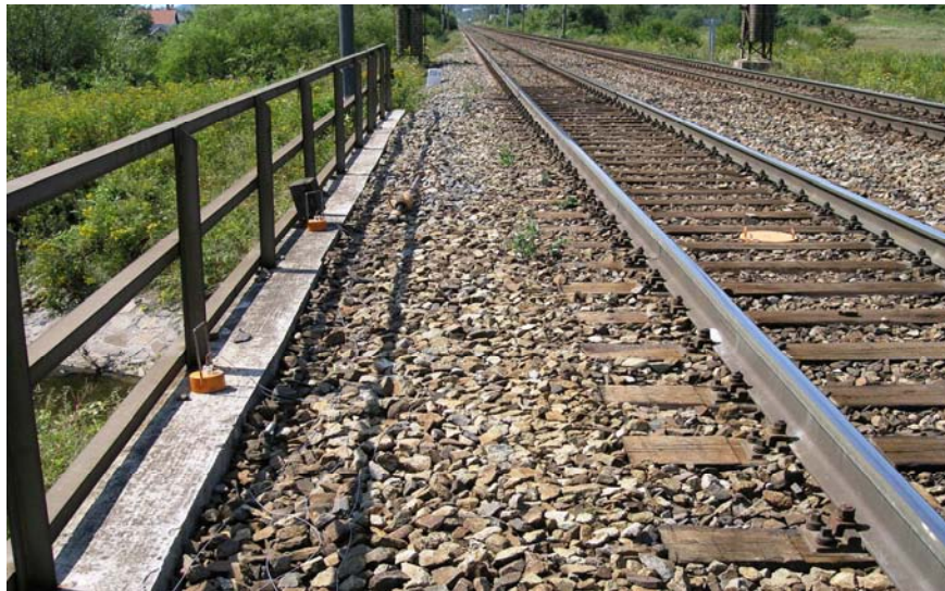
Fig. 7: Accelerometers with amplifiers – a part of CBMS
