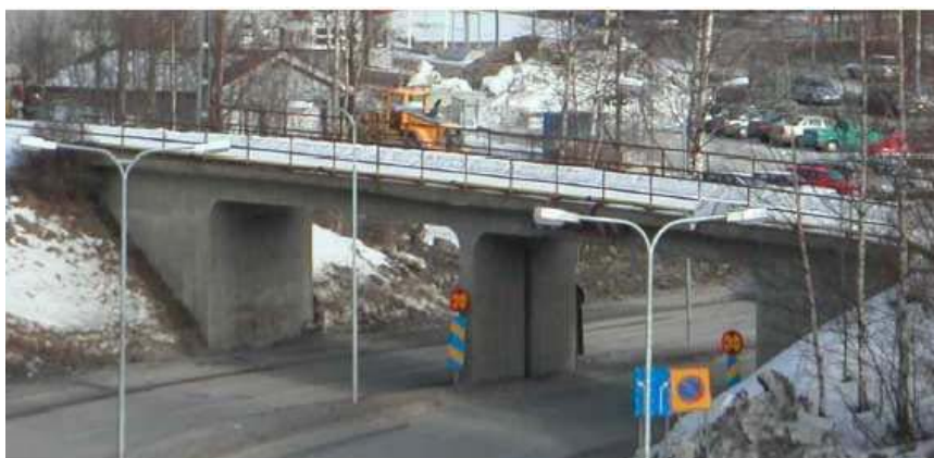
Fig. 1: Örnköldsvik Bridge (Elfgren et. al., 2007)
