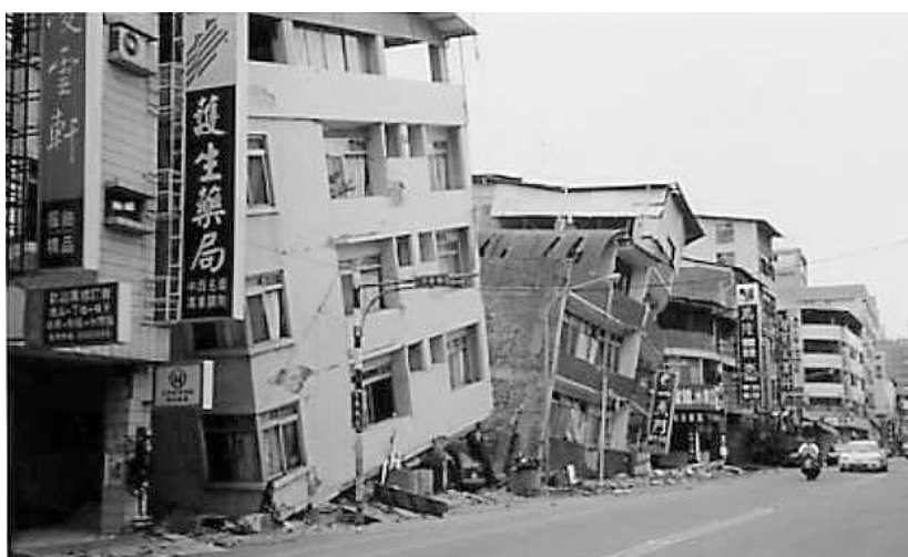
Fig. 1 Consequences of earthquake (Murty et al. 2001)
