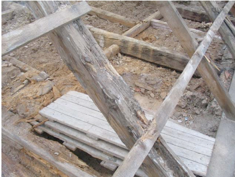
Fig. 1: View of the roof beam structure.
