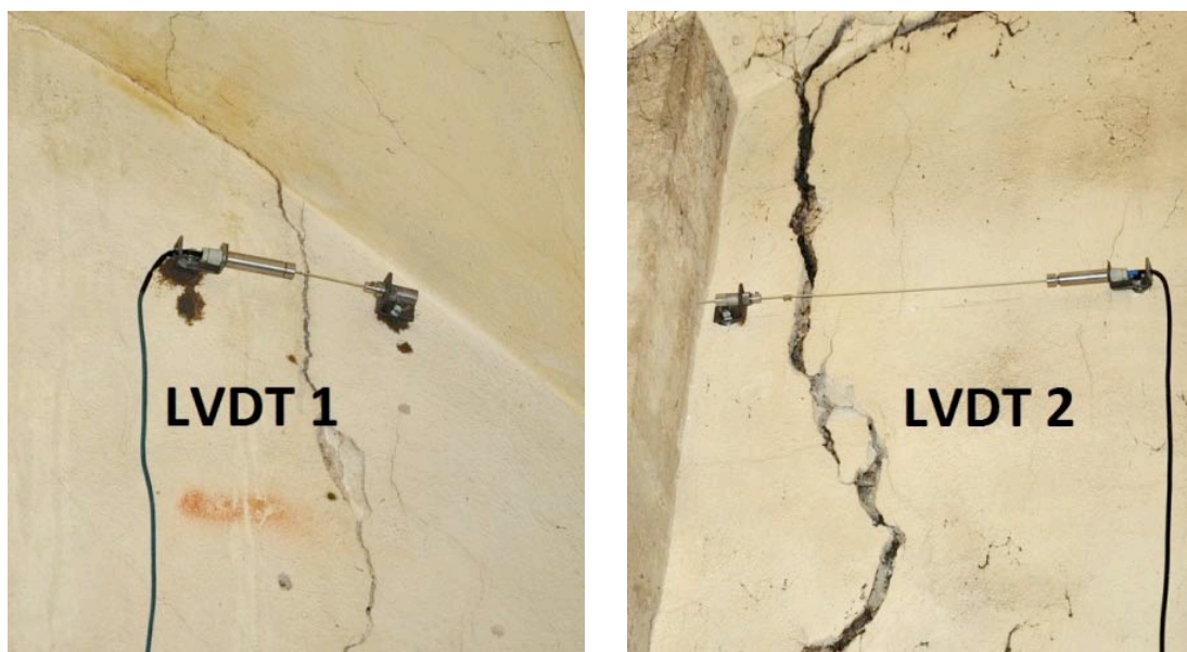
Fig. 10: LVDT set up, a) an inner side of the wall, b) an exterior side of the load-bearing wall
