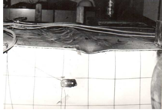
Fig. 12: Buckling of narrow flange at the gap of intermittent fillet welds
