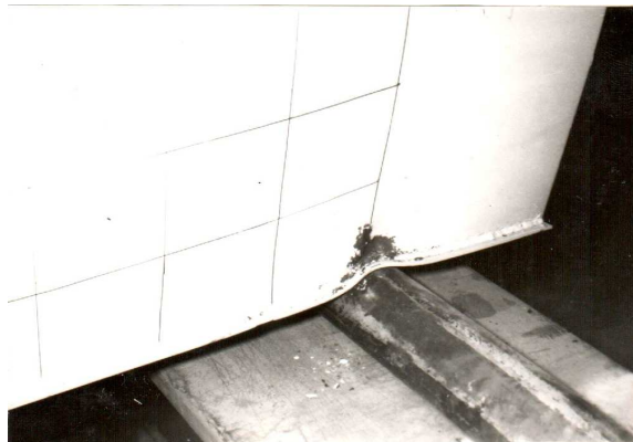
Fig. 4: Local crushing of the web at support
