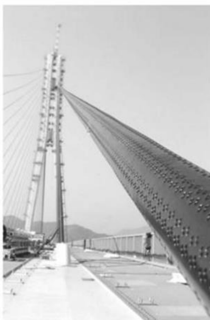
Fig. 5: The example of cable surface indentation used on the Tataru bridge
