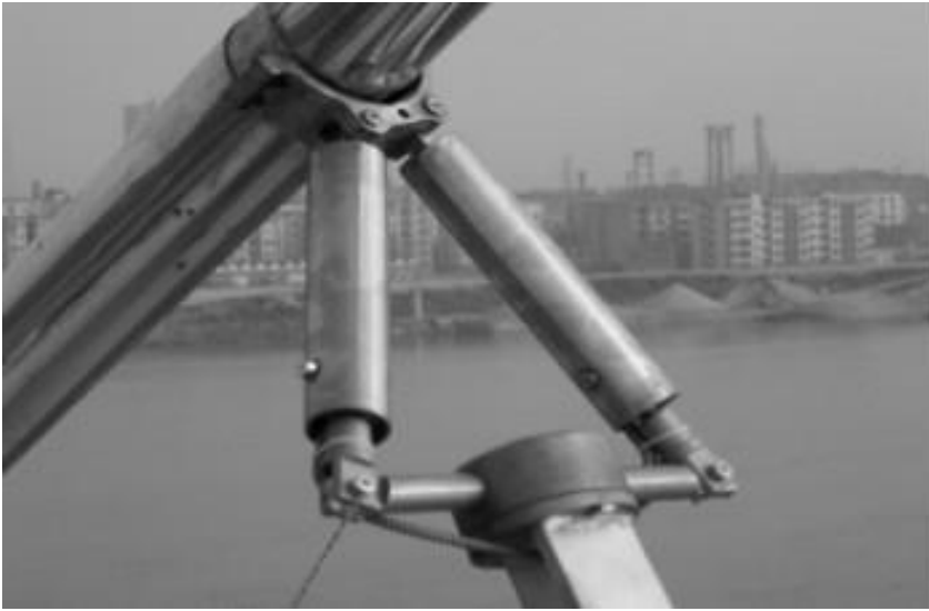
Fig. 9: An MR damper installed in the Doingting Lake bridge.
