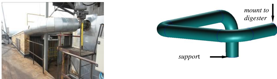
Fig. 2: The upper pipe section mounted to the digester.
