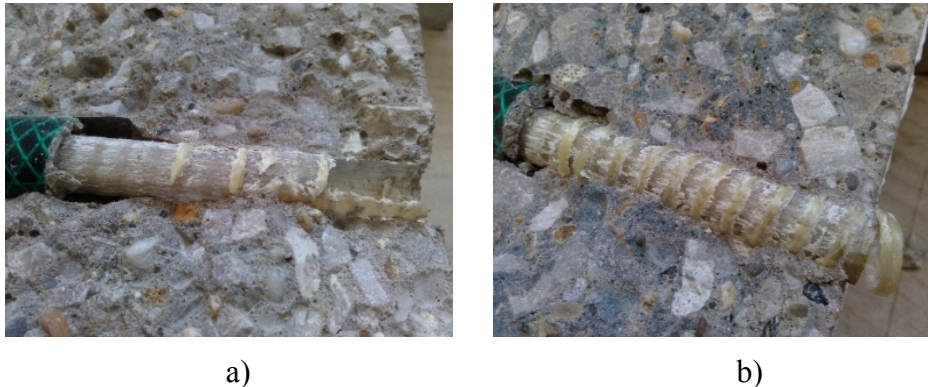
Fig. 3: The test sample failure a) 3 days after concreting, b) 28 days after concreting
