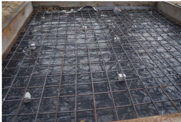
Fig. 5: Reinforcement – steel mesh.
