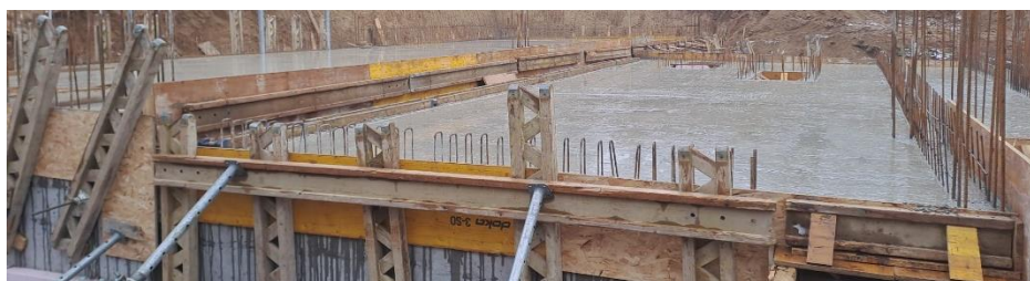
Fig. 2: Reinforced load-bearing slab made of recycled concrete (Trnava SK).
